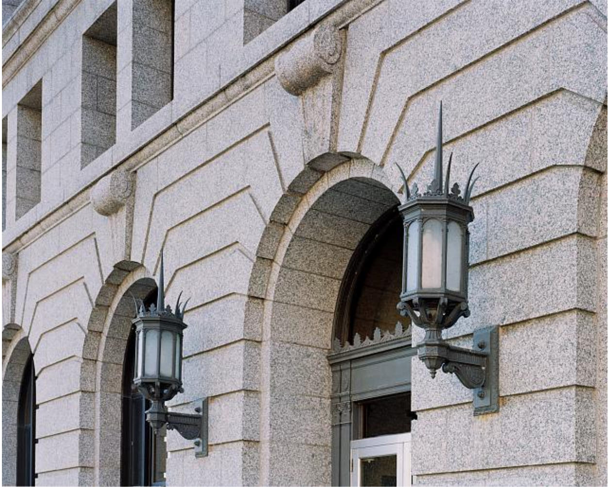
Front exterior detail of the Gerald W. Heaney Federal Building Duluth, Minnesota
